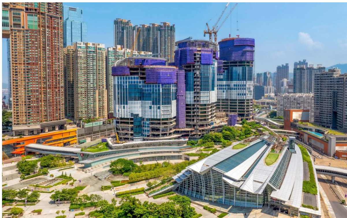
High Speed Rail West Kowloon Terminus Development International Gateway Centre (IGC) (office portion)
