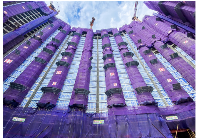
Metal scaffolding at our construction site in Kai Tak
