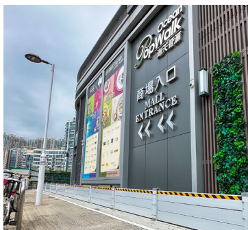
Floodgates installation at Ocean Pop Walk
