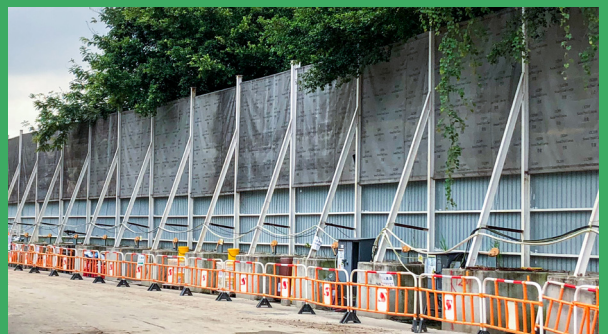
Wetland Seasons Park in construction stage
