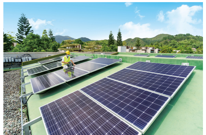
Valais - Residential development
