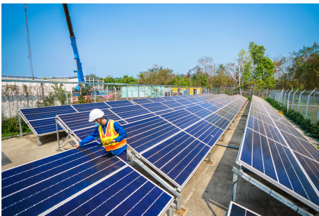
Construction site at Shap Sze Heung project
