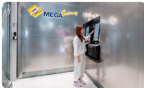
○ MEGA Gateway, SUNeVision's data centre in Tsuen Wan
