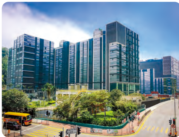
○ MEGA IDC, SUNeVision's new data centre in Tseung Kwan O
