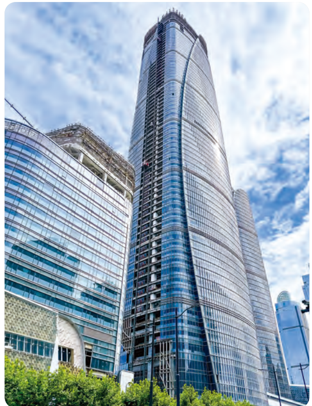
○ Tower B of Three ITC, Shanghai
