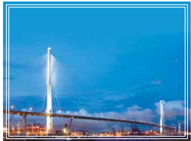
Stonecutter's Bridge is in the Tsing Sha control area in Hong Kong managed by the Wilson Group
