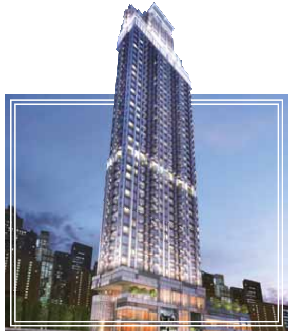
Modern exterior of Lime Stardom in Kowloon
