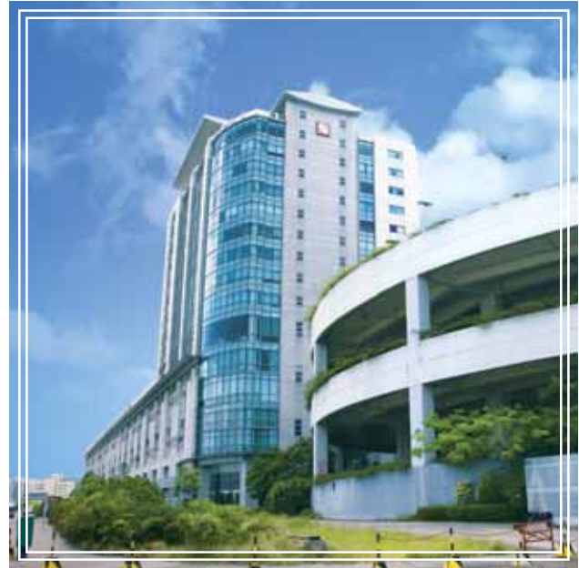
Quality service at the Airport Freight Forwarding Centre in Hong Kong attracts a global clientele
